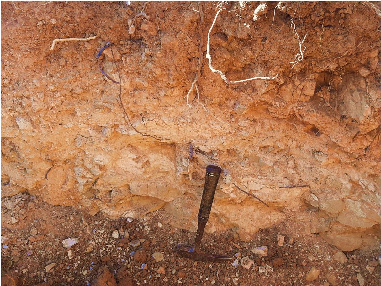
Figure 15. a 1 meter deep trench dug in the site shows a thick layer of soil and highly weathered rock underlying the area.
